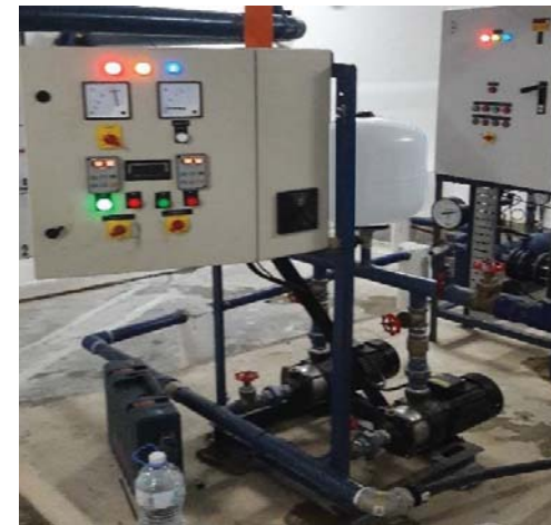
Variable Speed Transfer/Booster System - JMI-Simavis Horizontal Multistage Centrifugal Pump
