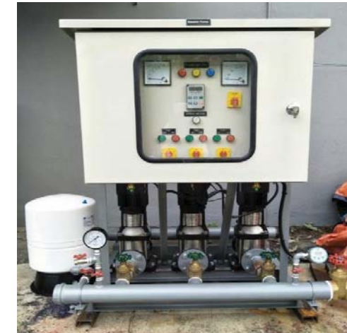
Variable Speed Transfer/Booster System - JMI-Simavis Vertical Multistage In-Line Centrifugal Pump
