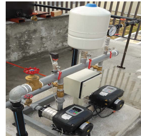
Variable Speed System (Single Phase Operation) JMI-Simavis Horizontal Multistage Centrifugal Pump
