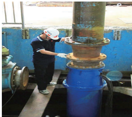
Pump Performance Test
