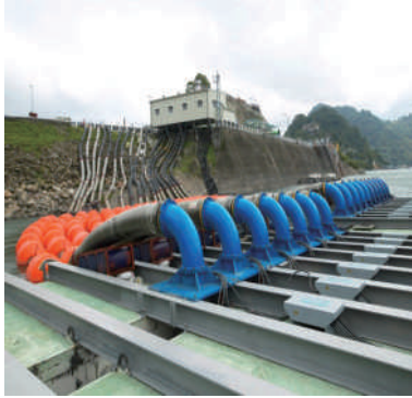
Water Intake at Reservoir
