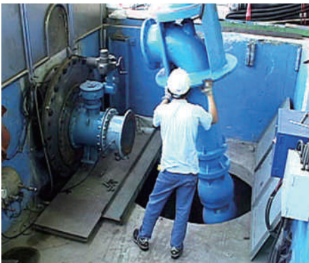
Pump Performance Test
