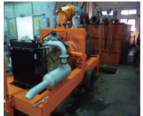
Pump Performance Test
